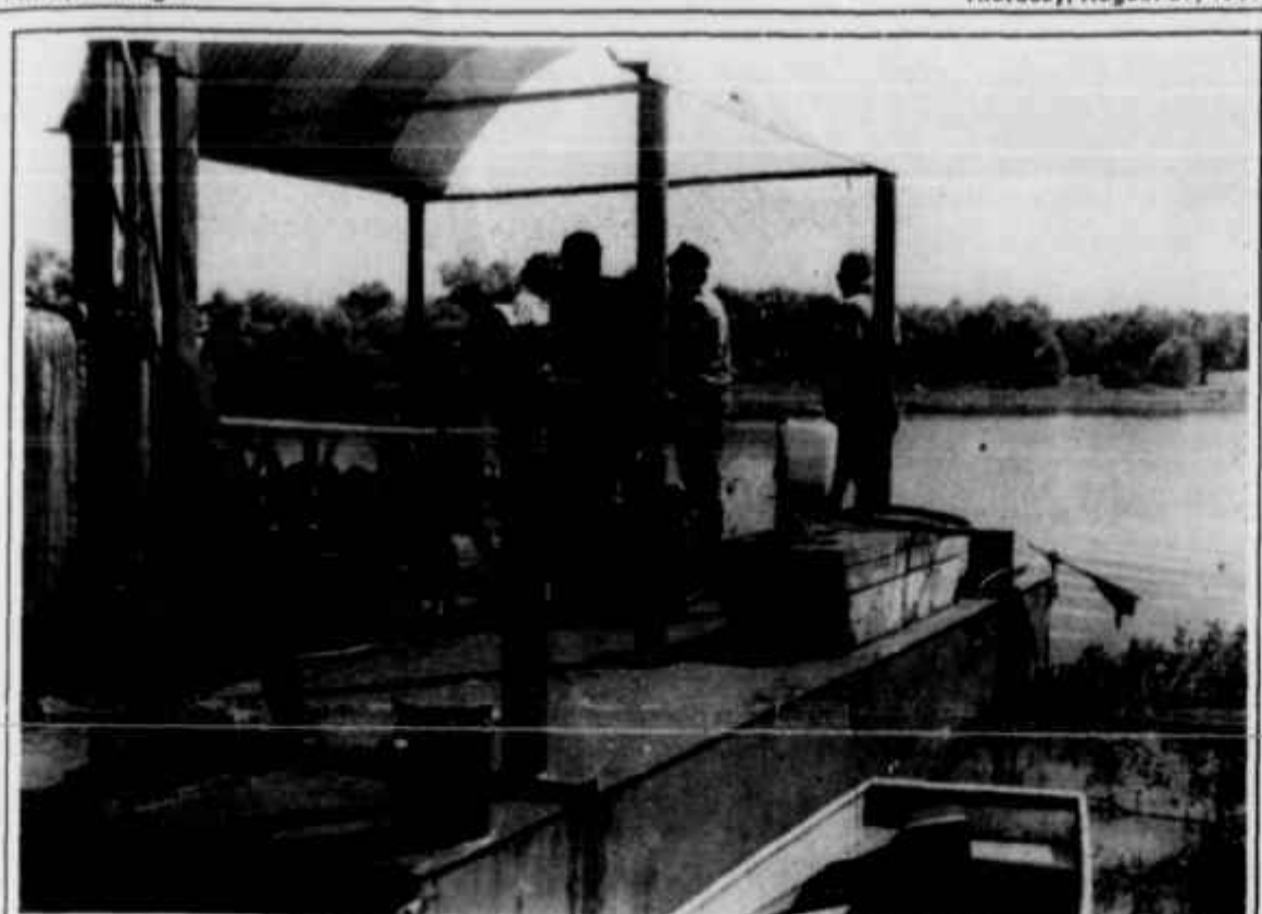
Dredging of McCreary Lake
